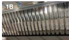
Grease-X-Tractor™ filters, first row of filters
