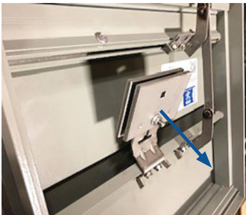
Figure 1: Bending counterbalance bracket away from blade towards the bottom (sill) of damper.
