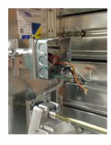
Mount the actuator to the actuator bracket assembly.
