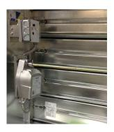
13. Drill holes in RRL (OCI and TOR) bracket (Item 4). Mount to the frame.
