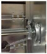
3. Loosen set screws on the actuator.
