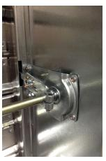
15. Attach the conduit, using the bracket, to the sleeve so it doesn't interfere with the blades.
