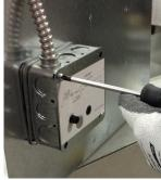
2. Disconnect the conduit from the sleeve.
