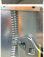
3. Loosen set screws on the actuator.
