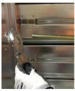
Loosen the bolt that holds the actuator to the bracket. Set aside the actuator and RRL (or RRL/OCI, TOR) assembly.
