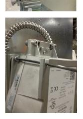
6. Take actuator bracket and standoff bracket off the sleeve.
