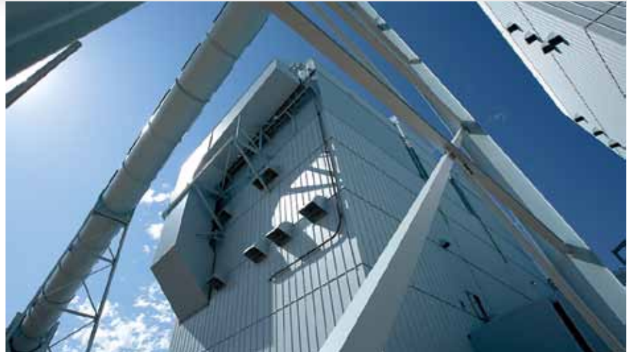
Basin Electric Air Quality Control building southeast corner.
