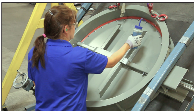
Seal Leakage Testing
