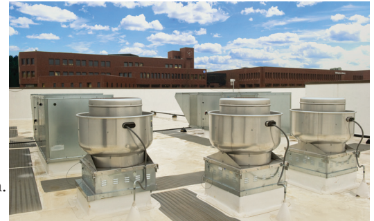
Greenheck spun aluminum upblast roof exhausters exhaust contaminated or grease laden air.
