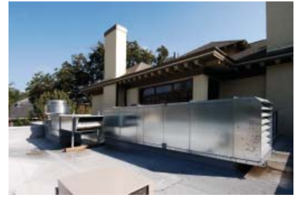
Greenheck's KSF supply fan, gas-fired make-up air unit, Model IGX, and CUBE exhaust fan.
