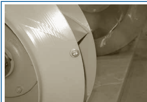
Permanently secured stainless steel bolts, nuts and washers used as balancing weights after paint
