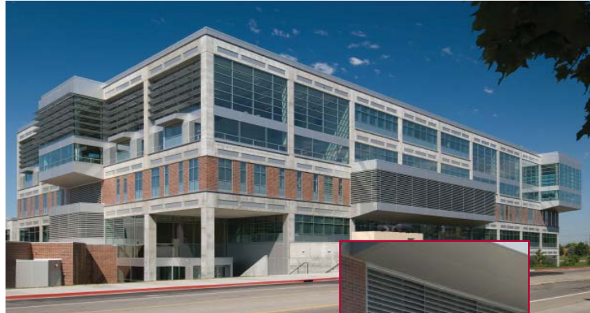
Two large custom air intake systems feature Greenheck louvers designed and manufactured to meet precise architectural specifications.
