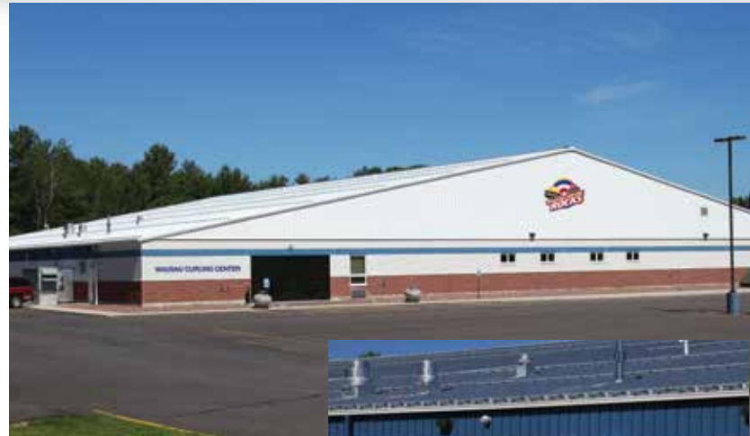
Top - Exterior view of Wausau Curling Center Right - Greenheck Rooftop Ventilator, Model RV
