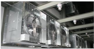
Greenheck's custom-designed special direct drive "Utility Duty" propeller fans in a 90" x 90" wall housing
