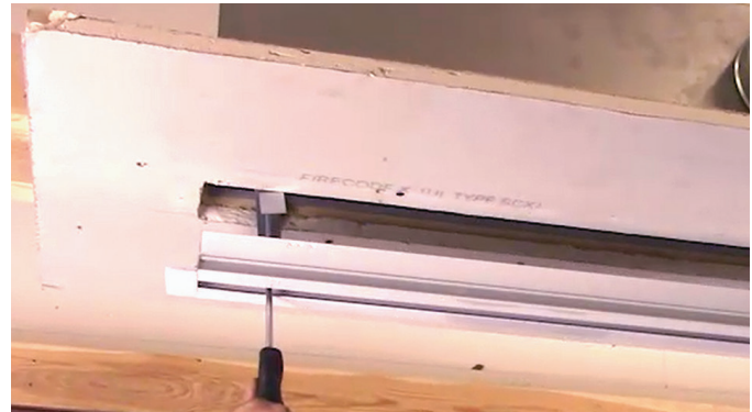
Figure 16 (Step 4B): Hanger Bracket Install Using Angles (other methods similar)
