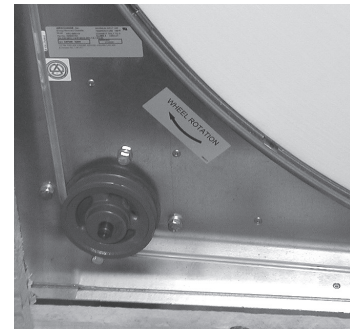
Wheel Belt & Pulley
